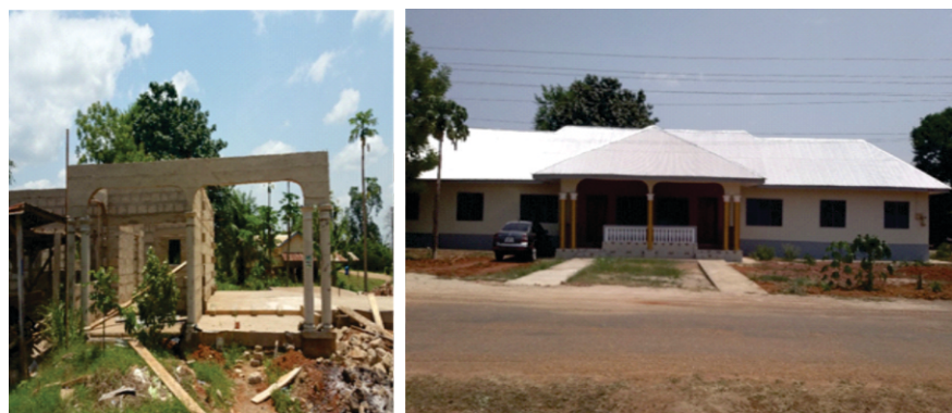
Figure 4: Previous and completion State of Doctors Bungalow 3
